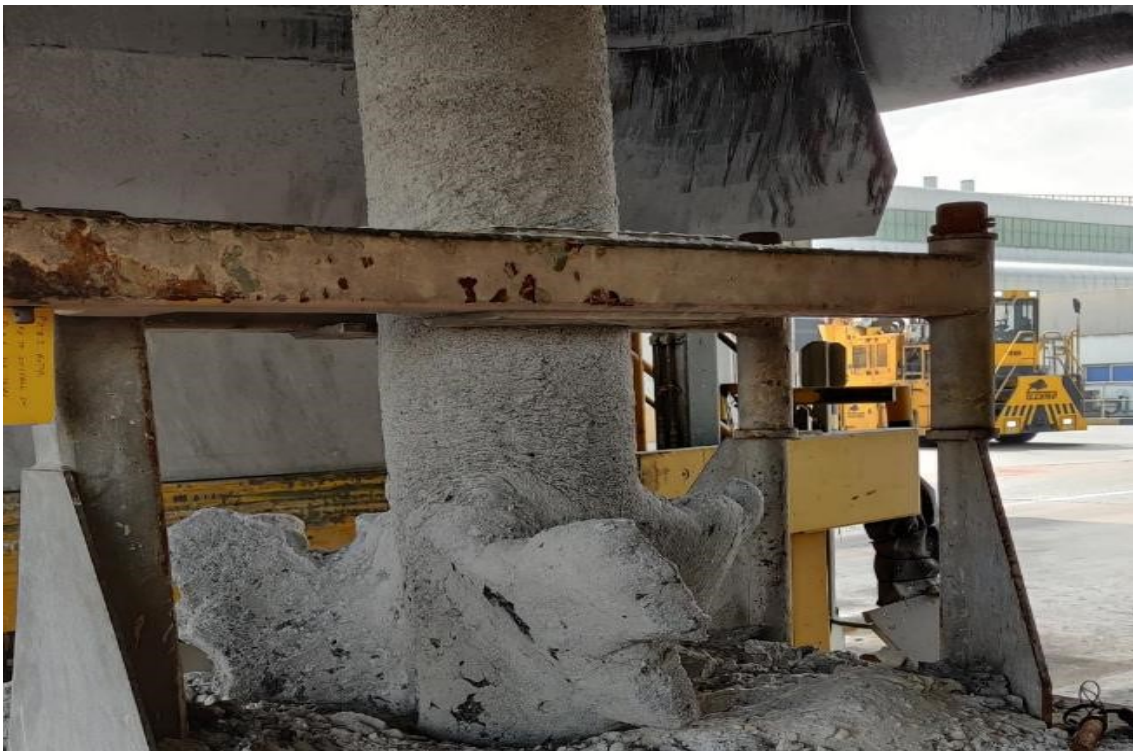
Figure 7. Condition of replaced rotor with eroded impeller blades.
